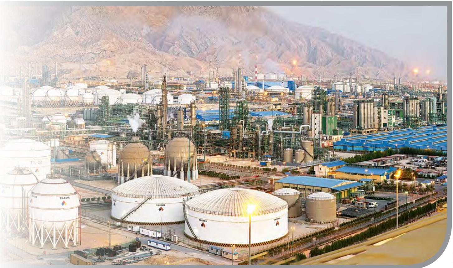
**HDPE unit****Licensor:** Lyondell Basell**Annual production capacity:** 300,000 MT**Feed:** Ethylene, hydrogen and butane**Number of grades:** 23**Products:** Small blow molding, large blow molding, stretched tape, monofilament, cable pipe (natural color) and film**Features**
